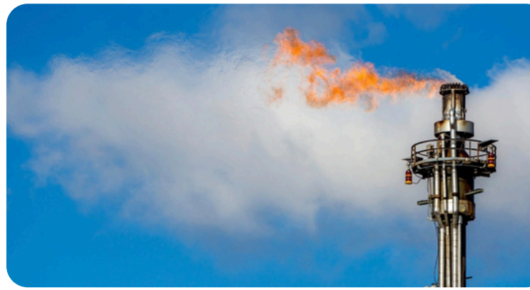
Pictured is a representation of a flare during use. Image used with permission courtesy of CleanAir.com/tag/flares/
